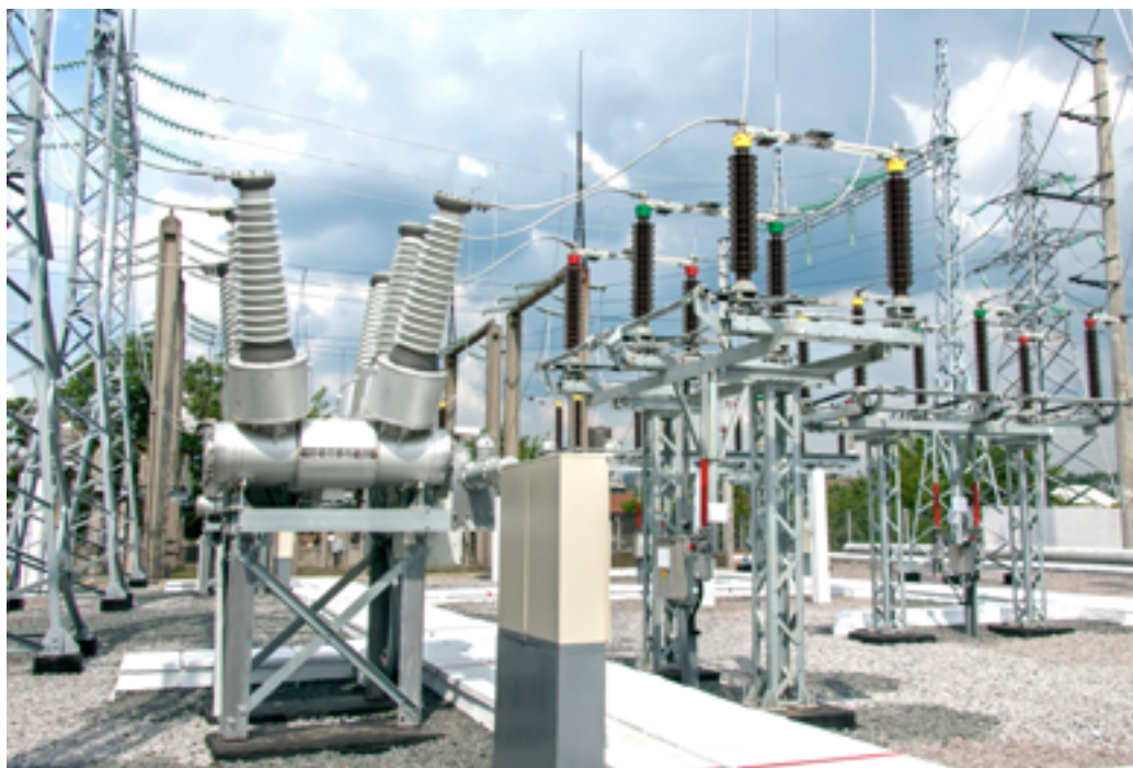
Figure 1: On-site medium voltage power distribution.
