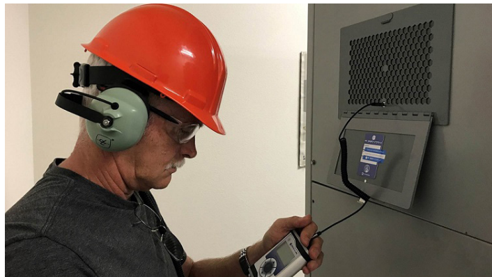
Figure 2: An inspector using an EMSD to collect Ultrasound Data. Source: IRISS
