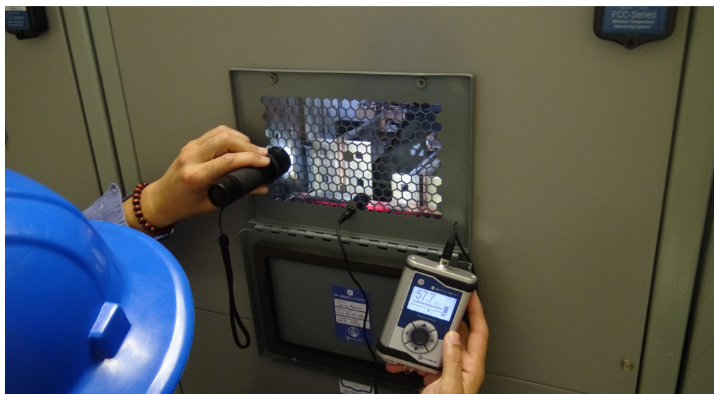
Figure 1: Electrical Maintenance Safety Devices can ease some of the physical burden of work on aging electricians by redesigning common tasks to be less hazardous and strenuous. Source: IRISS
