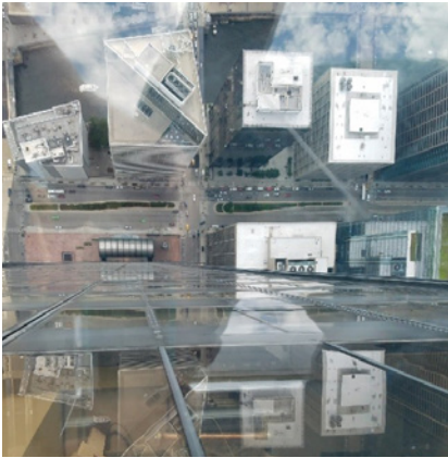
Figure 1: Looking down through the plexiglass box floor to the street below (Wacker) on the Skydeck at Willis Tower, Chicago. (Source: Paul Golata)
