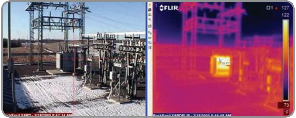
Figure 10. Visible light and IR images of a substation showing a transformer with excessive temperature.
