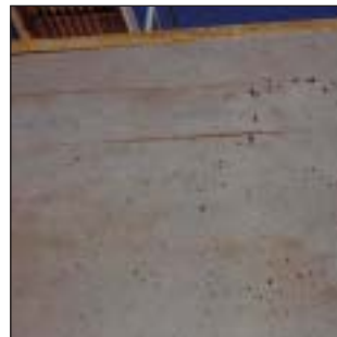
New concrete after abrasive blasting to remove laitance and expose bugholes
